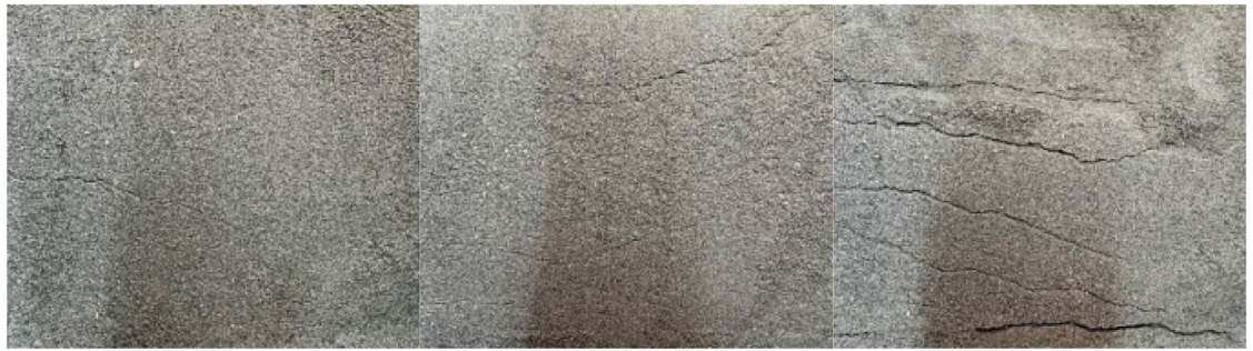
(a) Condition 1: Fracture development in the original reservoir area
