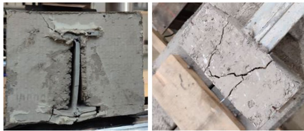
Figure 8. The typical failure of the support block of the first series beam.
