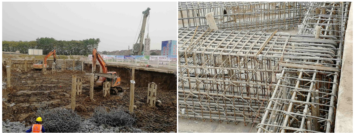
(a) Early construction
