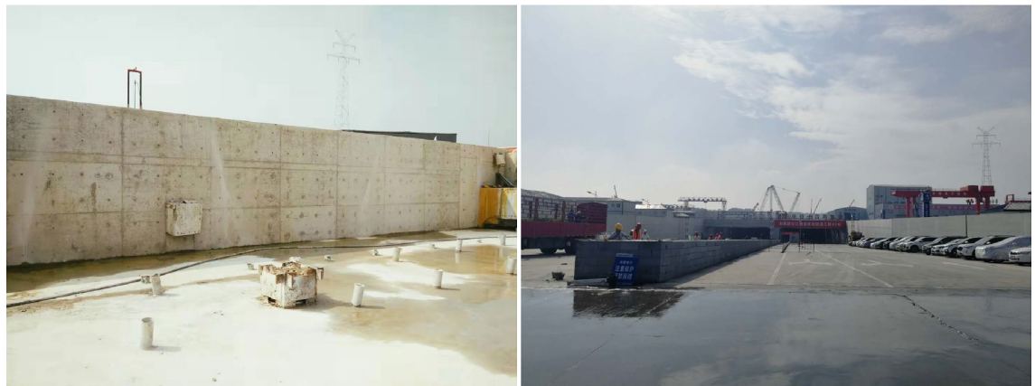
(e) Later construction
