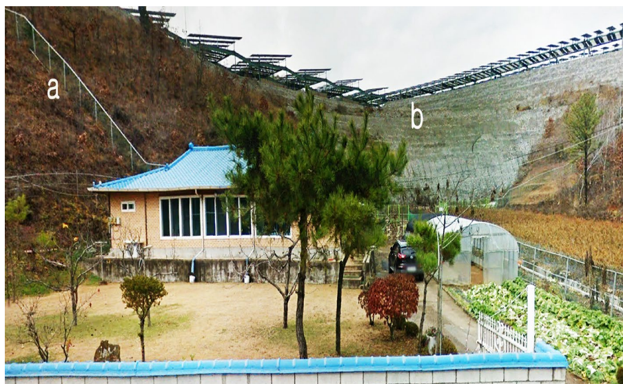
Figure 6. Typical scene of the agrophotovoltaic system observed in the experimental site, (a) a stair for farmers to access crops cultivated under solar panels, (b) cement-concrete structure converted from a mountainous landform. The fixed solar panel surroundings, captured from Google Earth street view, were obtained from Google Earth Pro 7.3.4 ( https://www.google.com/earth/versions/#earth-pro ). The image created in Google Earth Pro 7.3.4 and Adobe Photoshop CS3 ( https://adobe-photoshop-cs3-update.en.softonic.com/ ).
