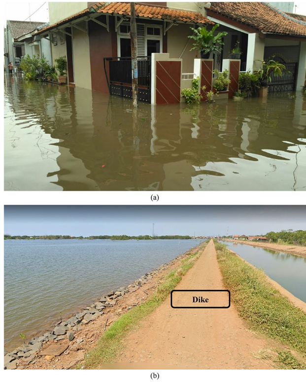
Figures 8. Flooded houses after tidal floods (a) 72 . A dike in the Pekalongan coastline (b) 73 .
