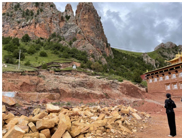
Figure 2. Panorama of the landslide.
