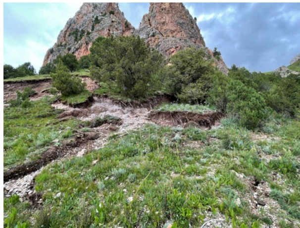
Figure 5. Landslide tensile cracks (2021.08).
