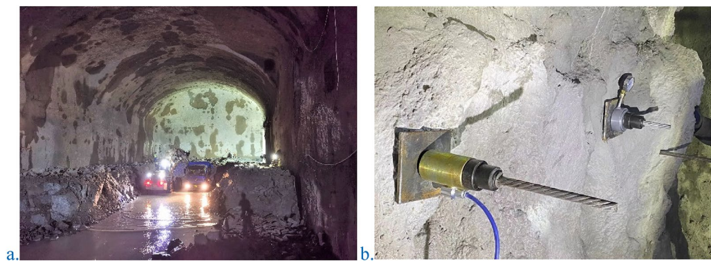
Figure 23. Real view of the tunnel.
