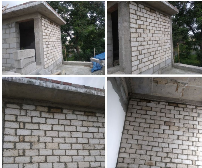
Figure 13. Prototype wall construction from gypsum-agro waste hollow blocks.
