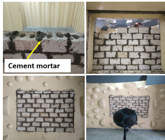
Figure 9. Test wall construction for sound transmission loss in the reverberation chamber.
