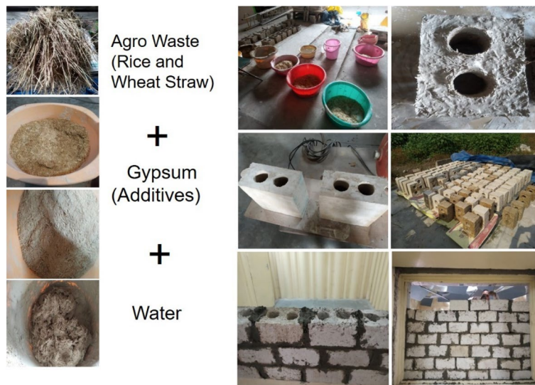
Figure 2. Process, casting, sun drying and wall construction of agro-waste gypsum blocks.
