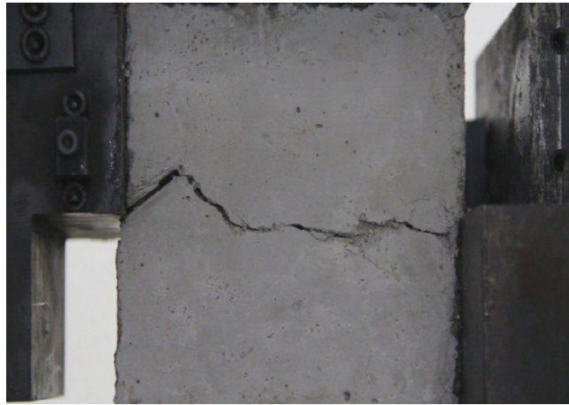
Figure 14. Photograph of a specimen showing fractures penetration.
