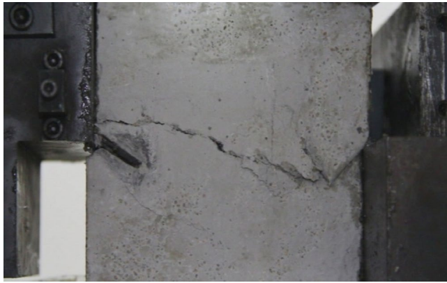
Figure 26. Photograph of a specimen showing fractures penetration.
