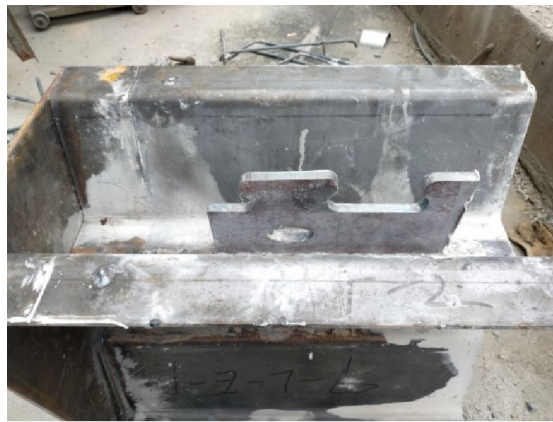
(a) Deformation of PZ shear connector
