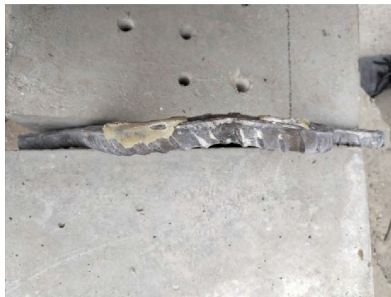
(b) Deformation of transversal reinforcement
