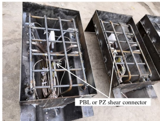
(b) Reinforcement of precast slab
