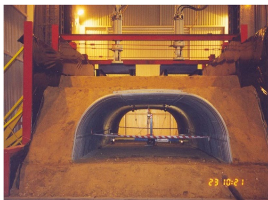
Figure 8. General view of the research model after soil backfill.
