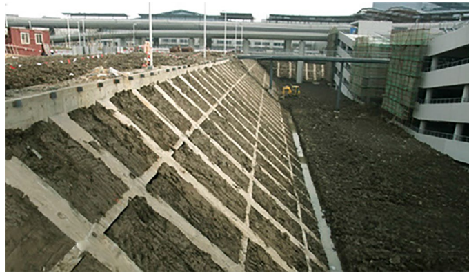
Figure 1. Frame protection of soil slope.
