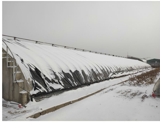
Figure 4. Field picture of greenhouse snow load.
