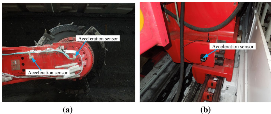
Figure 11. The installation position of the vibration acceleration sensor of the rocker arm and the walking box, for rocker arm (left) and drum (right) (a) and walking box (b).
