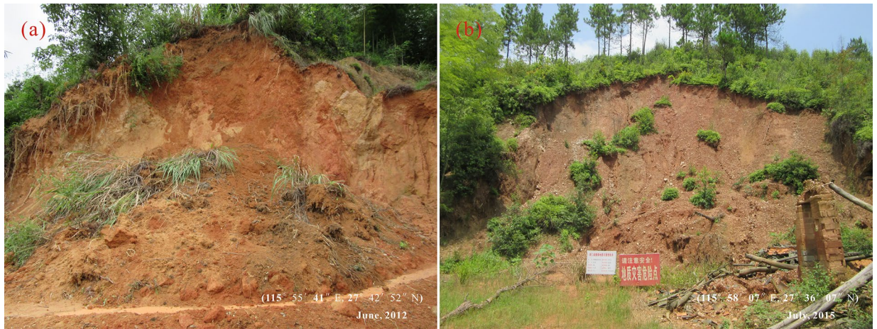
Figure 3. Photos of the rainfall triggered landslides in the study area.
