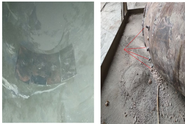
Figure 4. Samples installation inside the elbow.
