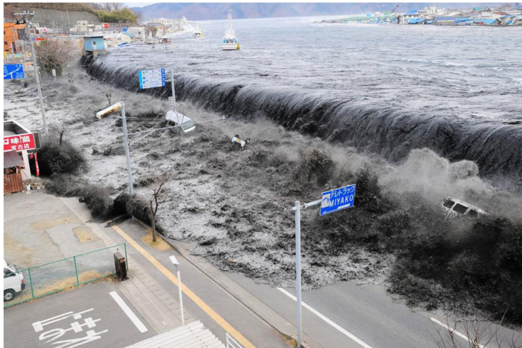
Figure 1. Tsunami overtopping a levee in Miyako City, Japan during the 2011 East Japan earthquake 26 .
