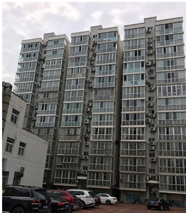
Fig. 1 Building appearance (south elevation).
