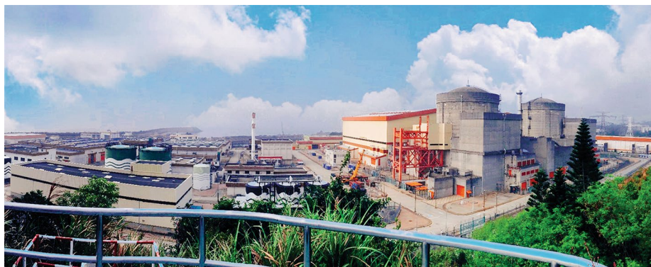
Dayawan nuclear power plant in China. Credit: Lei Huang, Wei Yu
