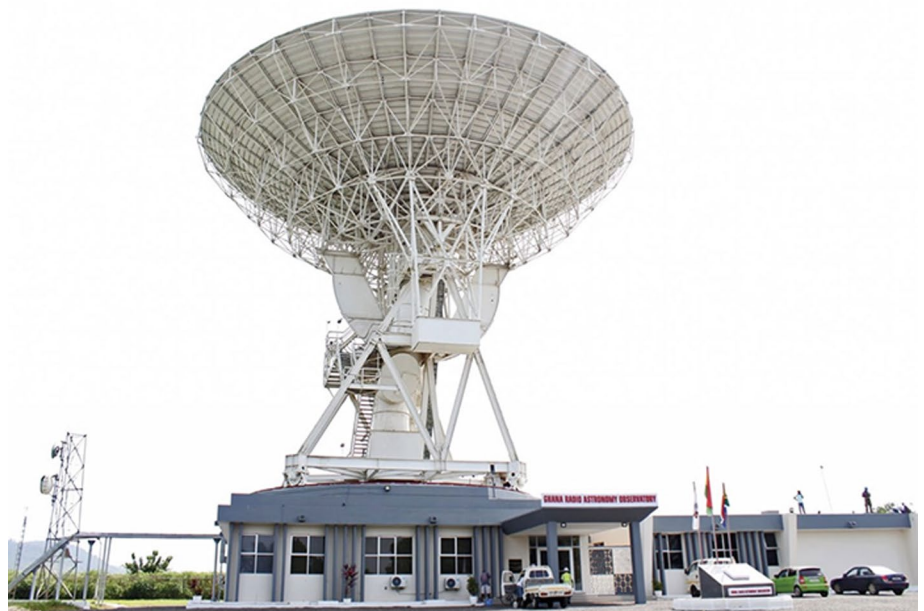
Fig. 1 | The 32-meter radio telescope at the Ghana Radio Astronomy Observatory. The dish was previously used as a satellite Earth station.
