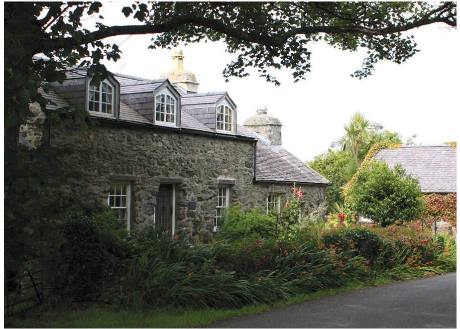
Fig. 6 The renovated cottage
