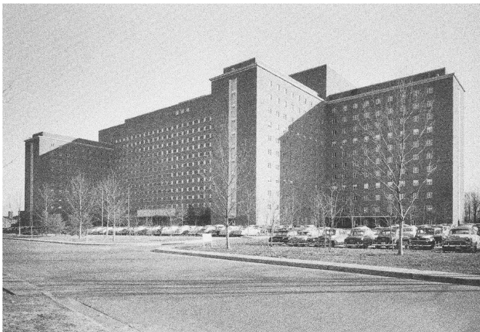
Figure 4. Building Ten (The Clinical Center) of the National Institutes of Health in the 1950s.
