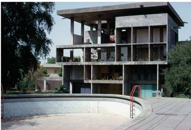
Figure 15 | Le Corbusier, Villa Shodhan, Ahmedabad, India 1951–1956 exterior, swimming pool, ca. 1965 exterior, detail of western façade, ca. 1965. Photograph by G. E. Kidder Smith. Source: image reproduced by permission of Massachusetts Institute of Technology. Copyright (© Massachusetts Institute of Technology, 2017). This figure is not covered by the Creative Commons Attribution 4.0 International license.
