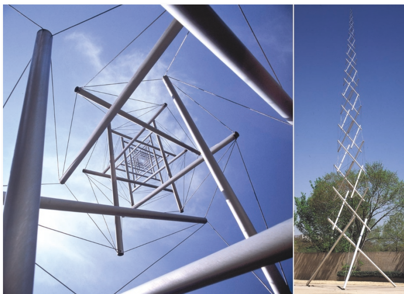
Figure 2 Interplay between compression and tension can stabilize structures at all length scales. The Needle tower by Kenneth Snelson is a macroscopic example of a structure in equilibrium between compression (aluminum tubes) and tension (steel cables), that leaves us with the puzzling impression of tubes floating in space. It is a similar construction principle that holds together some zeolitic frameworks.
