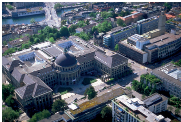
The impressive main building of ETH Zürich, a technical and scientific university in Switzerland.
