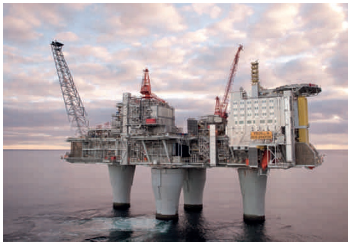
Statoil Troll A natural gas platform off the coast of Norway is a feat of engineering.
