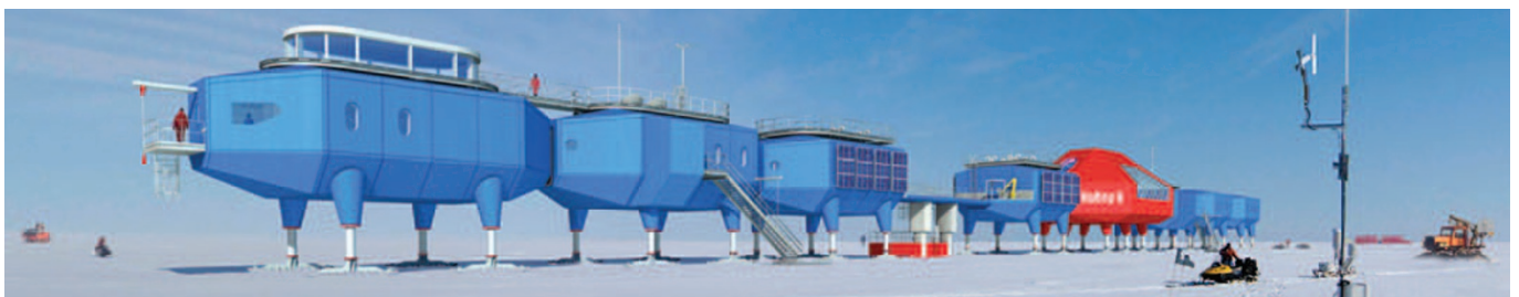
Home away from home. Artist's impression of the new British station Halley VI. Eight individual modules are mounted on hydraulic legs on skis to facilitate relocation.
