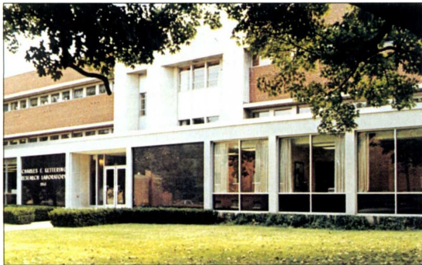
The Kettering Lab, which Battelle is acquiring.
