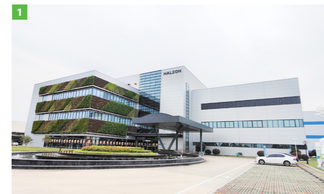
▲ 1. Haleon Suzhou Technical Center in Suzhou, China is one of the company's three R&D centres.
