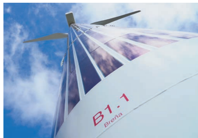
▲ A photodetector based on fullerenes (left) could be integrated in smartphones and enhance their security by turning the whole screen into a fingerprint reader. The curved surface of a wind-turbine pole (right) is covered with solar cells that incorporate fullerenes.
