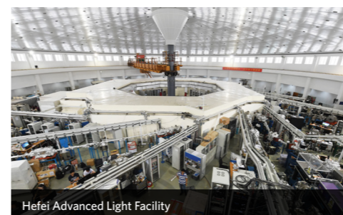
Hefei Advanced Light Facility
