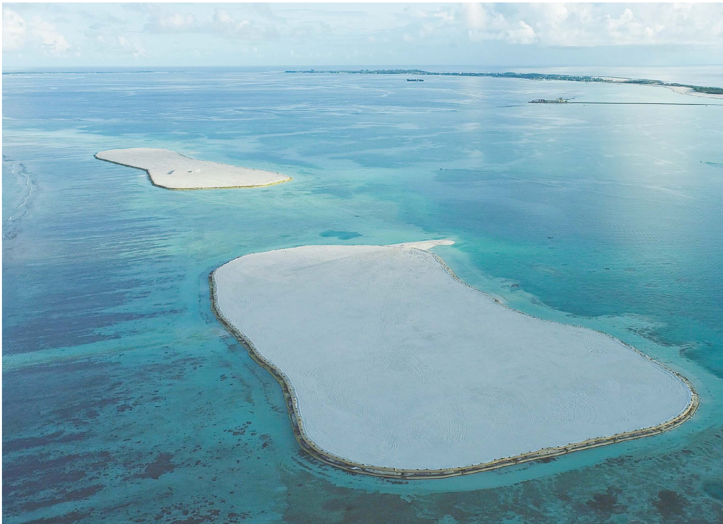
Artificial islands were constructed inside the lagoon of Addu Atoll in the Maldives to create space for new resorts.
