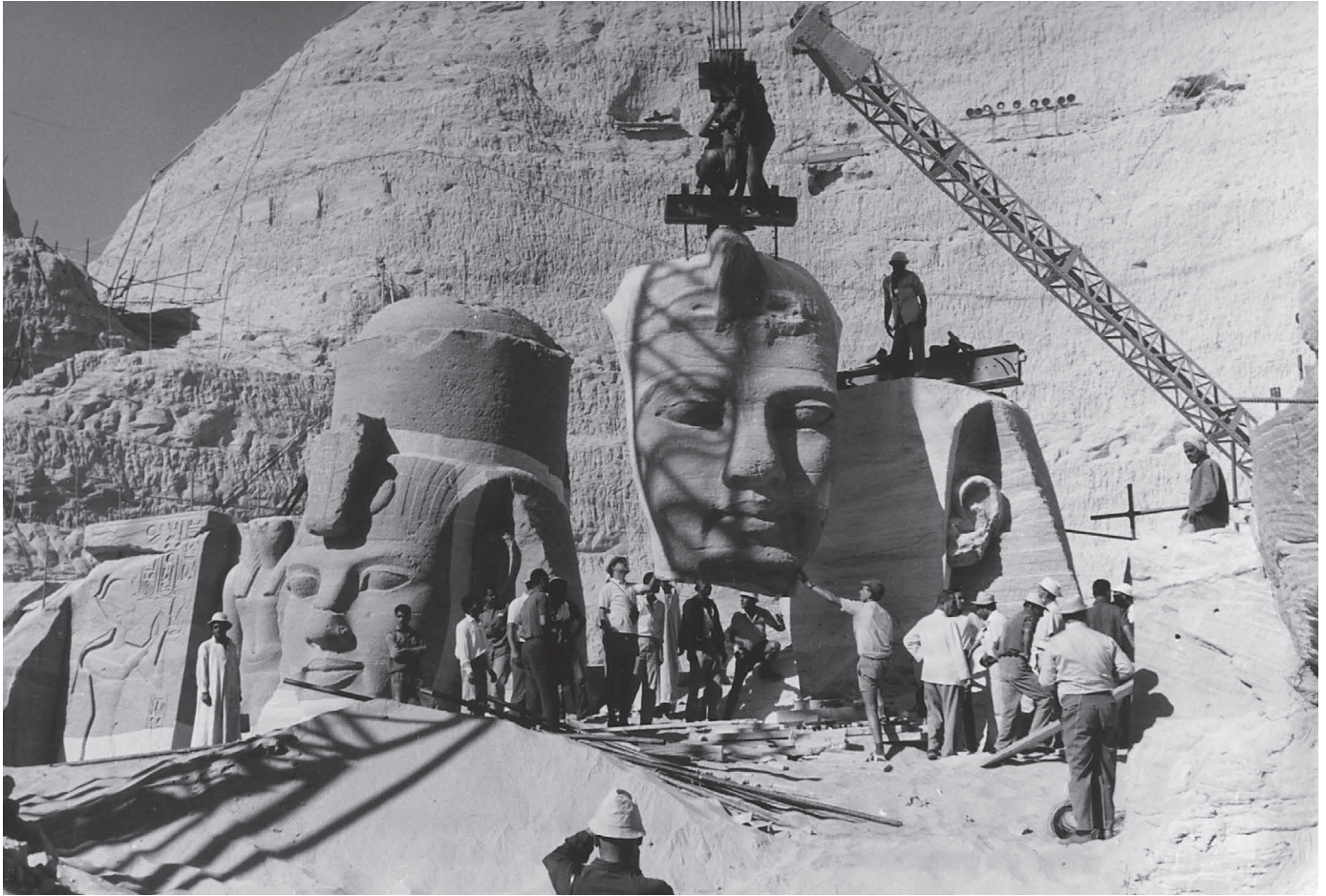
Workers move part of a statue during the relocation of the Abu Simbel temples in Egypt in the 1960s.
