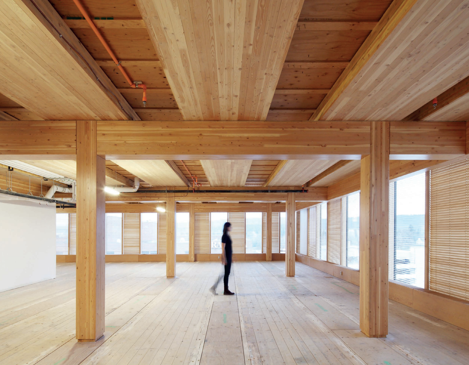
Canada's Wood Innovation and Design Centre has an entirely wooden structure, showcasing the potential for high-rise wooden buildings that lock up carbon.
