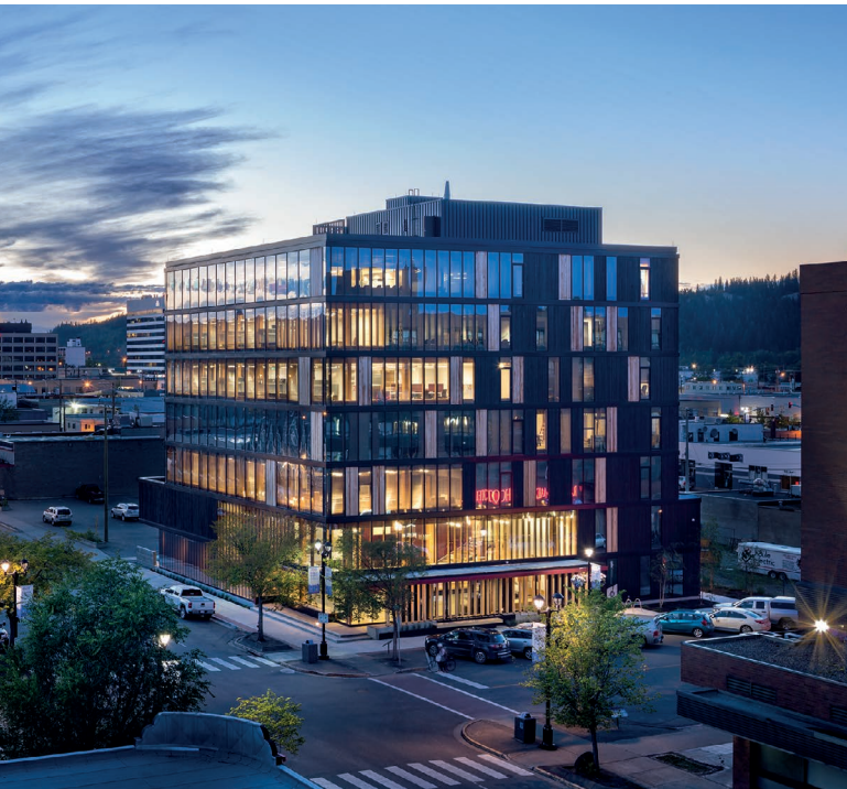
The centre's exterior was inspired by bark peeling from a tree trunk.
