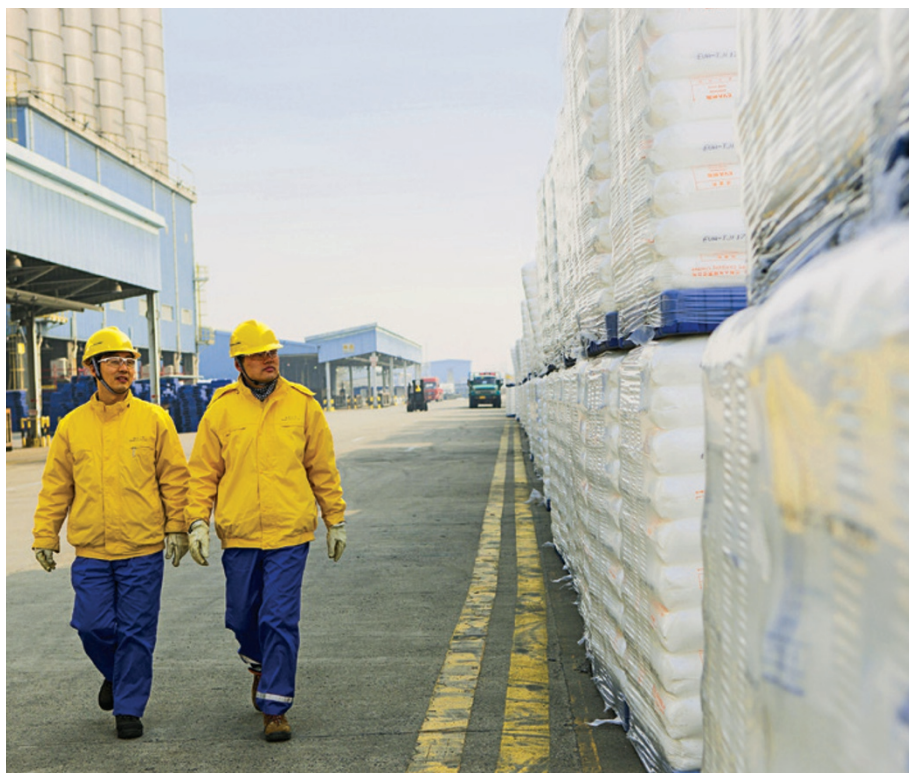
BASF-YPC Company's low-density polyethylene plant produces 400,000 metric tons a year.
