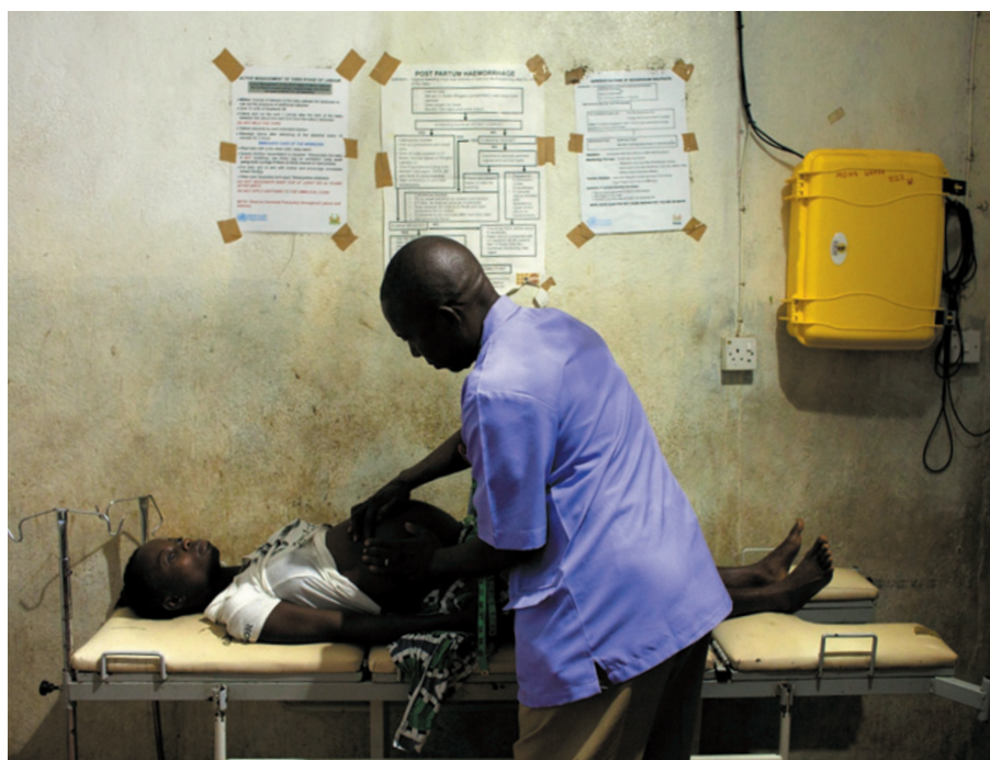
A wall-mounted 'solar suitcase' delivers power to a clinic in Sierra Leone.
