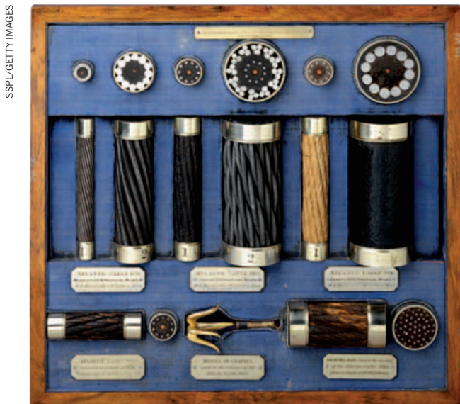
Sections of the Atlantic cables from 1858, 1865 and 1866.
