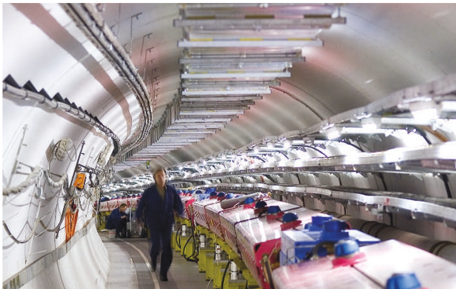
Massive project: the CERN particle-physics lab will beam neutrinos to Italy to see if they have mass.
