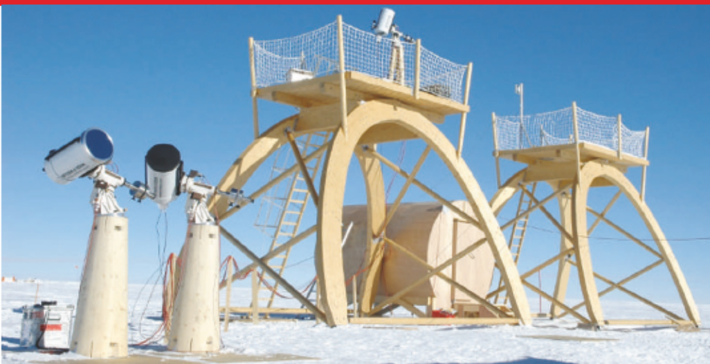
Reaching for the stars: the telescope platforms at Concordia were modelled on the Eiffel Tower.
