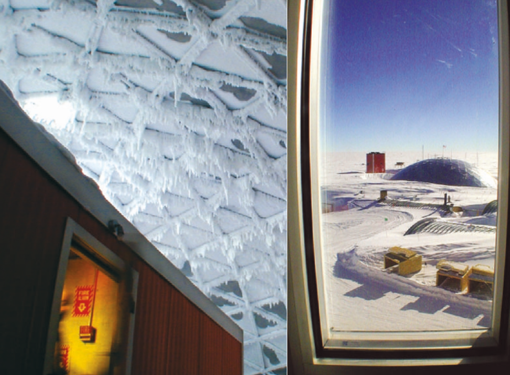
Halley V (left) risks being washed away, and the South Pole Station (middle, right) is drowning in ice.
