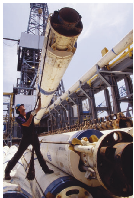
Figure 1 Acid attack: drill pipes on oil rigs suffer corrosion.
