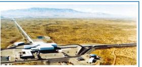
Washington state (see picture), and in Livingston, Louisiana (so that a detection at one site can be validated by a similar detection at the other). The two arms of each interferometer are 4 km long, containing vacuum tubes that are 1.2 m in diameter. The central building, where the arms meet, houses lasers and control equipment.
