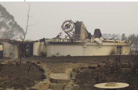
Gutted: the charred remains of Mount Stromlo Observatory — remarkably, some data survived.
