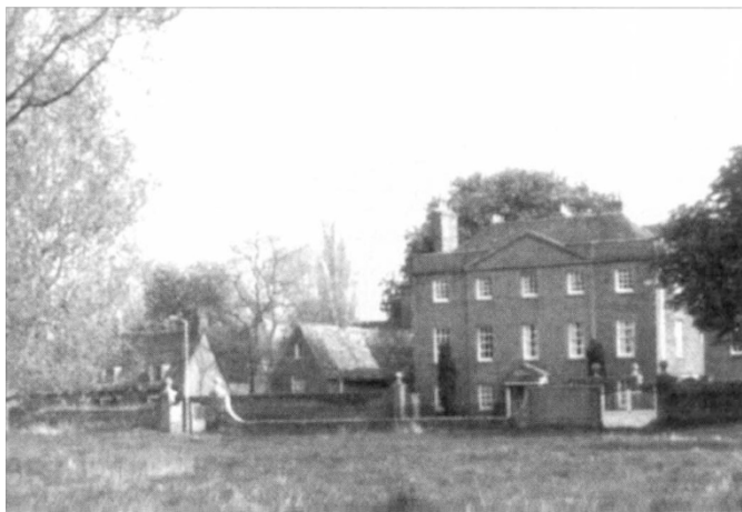
Farm Hall as it looked in March 1987.
