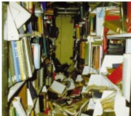
After the flood: around 380,000 volumes from the library at Colorado State University have been sent for recovery following the flash flood that breached a basement wall of the Morgan Library.
