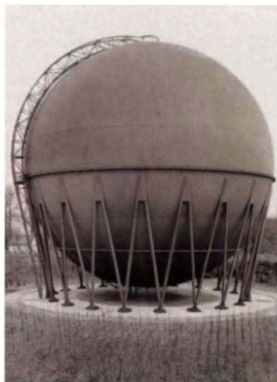
WHAT a gas — three types of gas tanks (or gasometers). The oldest is the multiple section type (left). It works on the same principle as a bell jar upside down in a tank of water. Spherical gas tanks store
