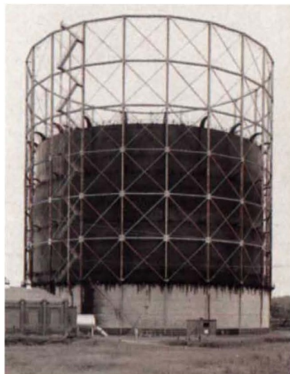
WHAT a gas — three types of gas tanks (or gasometers). The oldest is the multiple section type (left). It works on the same principle as a bell jar upside down in a tank of water. Spherical gas tanks store
