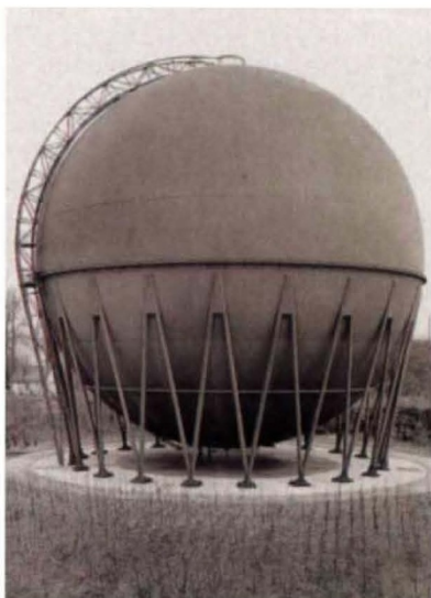
WHAT a gas — three types of gas tanks (or gasometers). The oldest is the multiple section type (left). It works on the same principle as a bell jar upside down in a tank of water. Spherical gas tanks store
