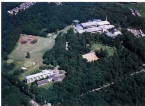
Aerial view of the Sagami centre.
