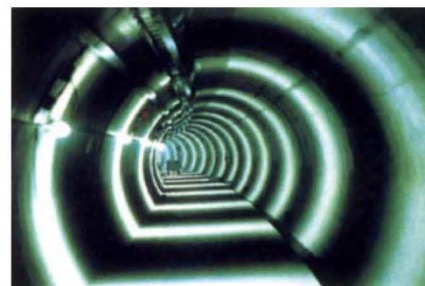
Driven round the bend: the LEP tunnel during the construction phase, before tidal effects had been considered.
