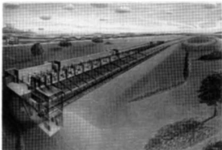
The linear accelerator is the first of four machines that will prepare protons for the SSC.
